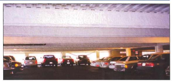
Protek-13<sup>th</sup> provides a brighter, safer work environment while protecting the fibrous insulation underneath from physical abuse.
